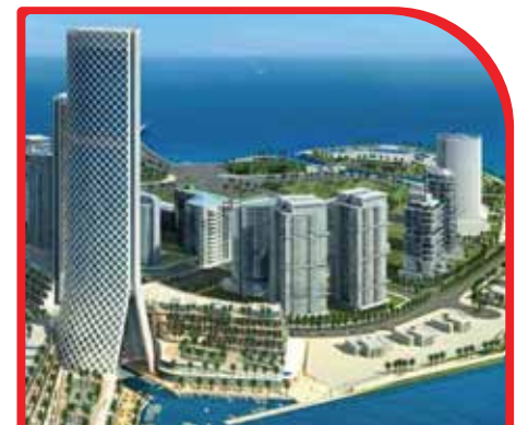
TAMEER TOWERS DUBAI, UAE
