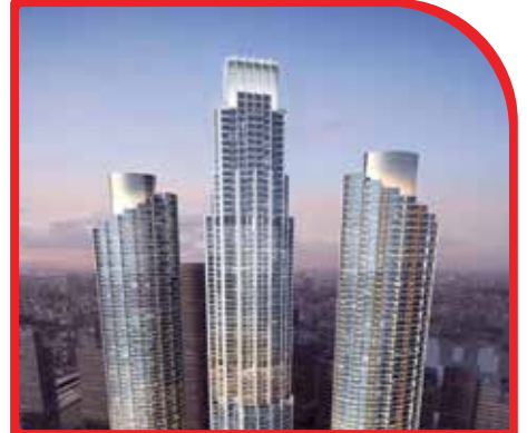
FOUNTAIN VIEW DUBAI, UAE
